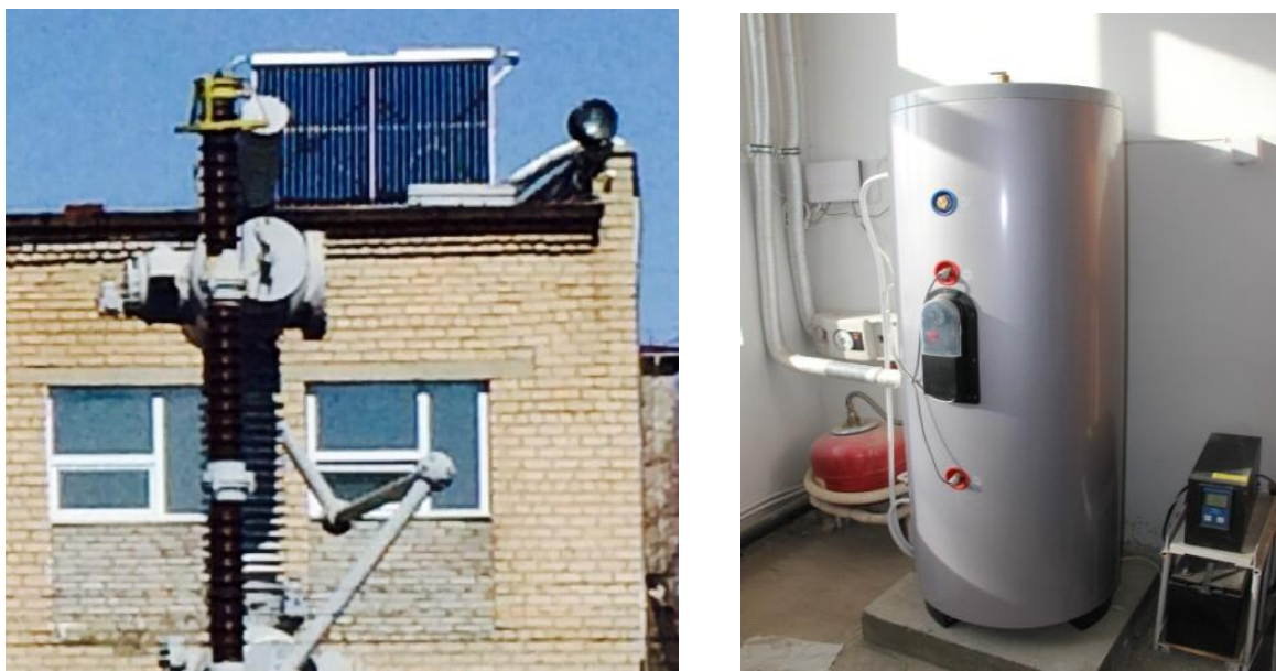
Figure 1.9 - Thermal solar collectors for heating closed water
