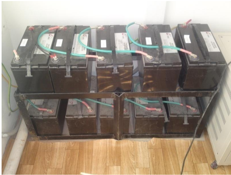
Figure 3.5 - Assembling the batteries of the wind generator.
